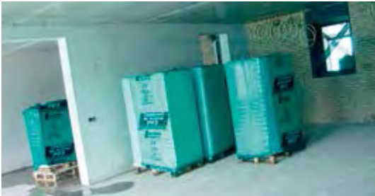
Conditions de stockage Photo: Lafarge-Gypsum
